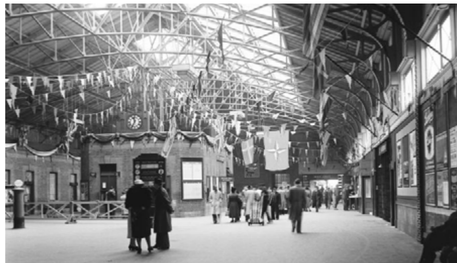
Figure 5.24 Tilbury Riverside Station Sources: https://nationalrailwaymuseum.wordpress.com/2012/05/29/celebrating-the-jubilee-royal-photos-from-our-archives/tilbury-riverside-station-1950-2/
