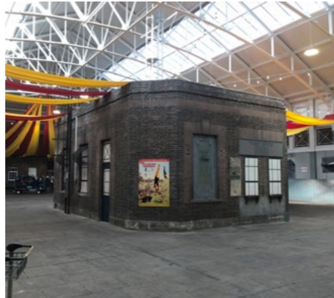
Figure 5.22 The Tilbury Riverside Station Building - Site Image
