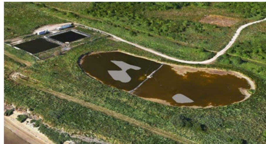
Figure 3.47 Broadness Water Treatment Facility and Leachate Treatment Plant
